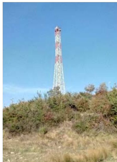
Figure 1 - The torch of an oil extraction site dominating the countryside. Suspicious flames have been reported by the residents - Corleto, October 2020
